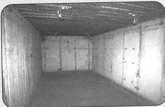
One of four crew sleeping quarters with three tier bunks
