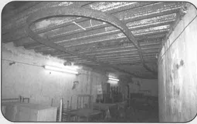
Shell magazine hoist rail above the school clutter
