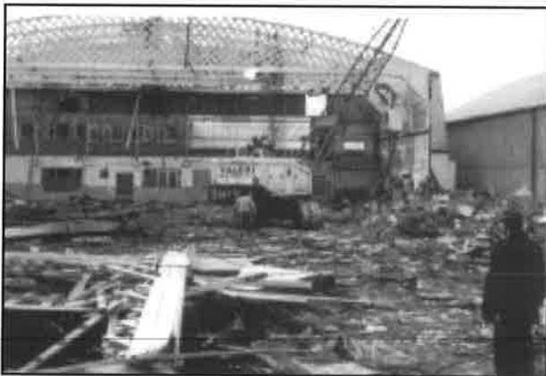
The General Service Shed being demolished circa 1970.
